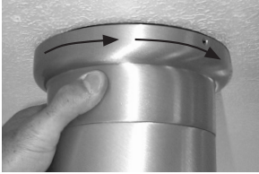
mount fan to plate
